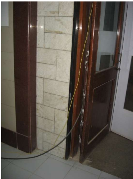
Look at these loose connections going thru doors.
